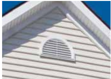
Half Round Gable Vent on vinyl surface
